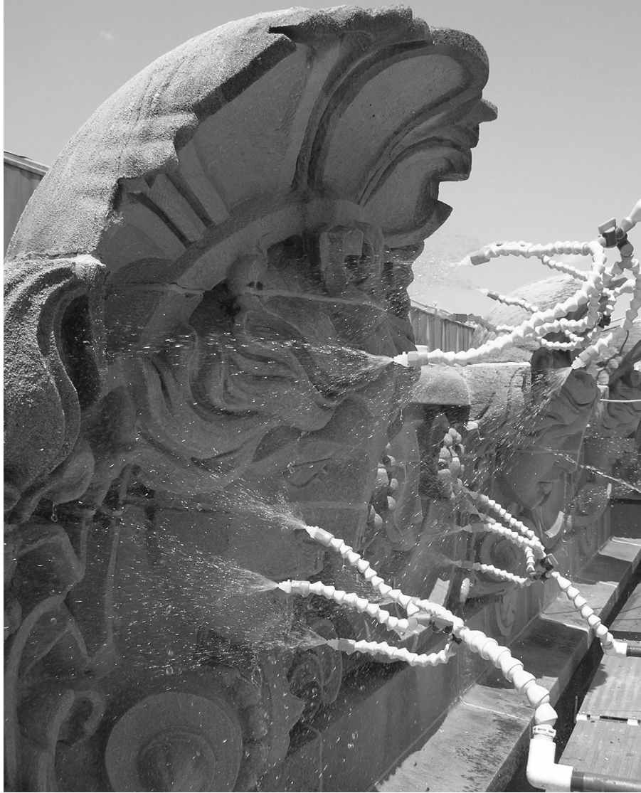
Figure 2 For very fine mist cleaning, adjustable nozzles are conformed to reach many areas of delicate stone crevices. Each nozzle is equipped with an arm that can be adjusted to reach difficult areas of access where soot and carbon build-up can occur.
