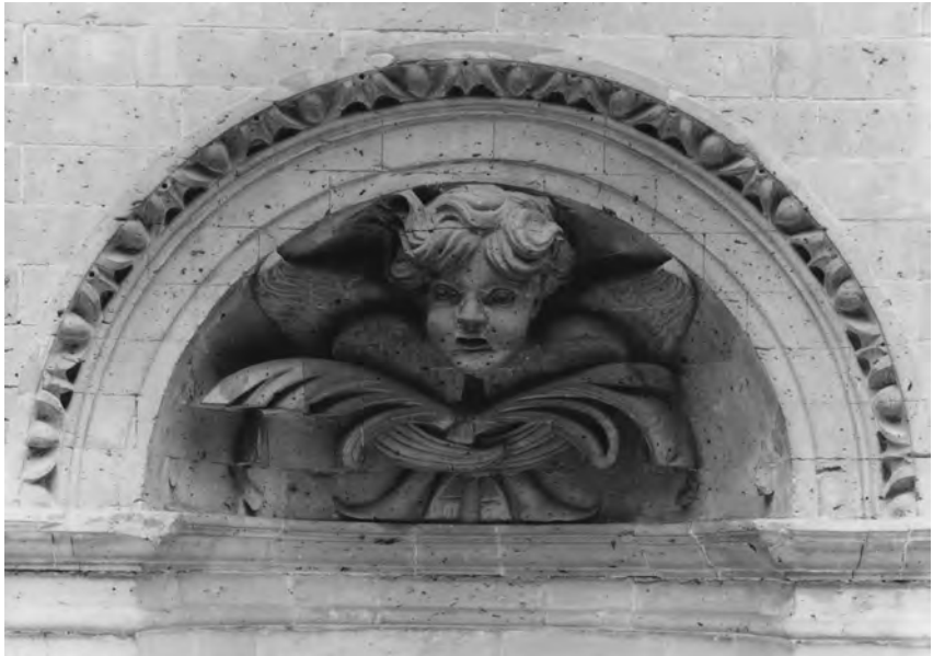
Figure 5.3 An excellent example of seventeenth-century gauged work: the head and wings of a cherub, or ‘Amorini’, in the hood of a niche, surmounted by an egg and dart label course. The carving is from a window pediment originally from a house in Enfield (d.1675) and now in the Victoria and Albert Museum, London. (Board of Trustees of the Victoria and Albert Museum)
