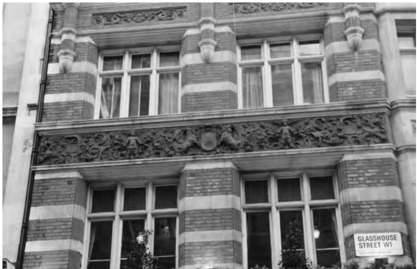
Figure 5.1 A very fine example of a carved gauged brick frieze on a public house in Glasshouse. (F. Lynch)
