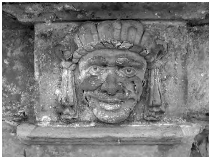
Figure 9.3 A delicately carved eighteenth-century Chilmark limestone mask head, from the façade of Longford Castle, Wiltshire. Facial features have become distorted due to the formation and exfoliation of gypsum skins.
