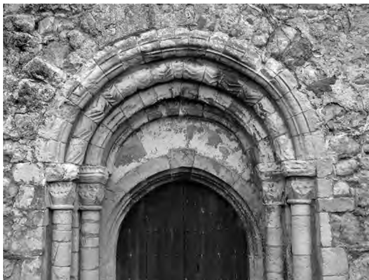
Figure 9.2 A fine twelfth-century west doorway carved in Caen limestone from Normandy, at Ruckinge Church, Kent. The stone exhibits signs of sulphation decay, and soot crusts are collecting in sheltered areas.
