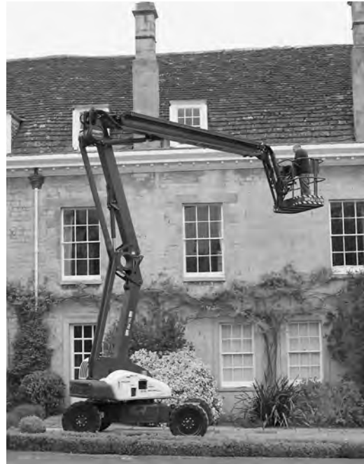
Figure 5.1b Powered-access platform used for inspection and maintenance tasks to chimney stacks and rainwater goods. With a maximum working height of 21.2 m, unrestricted working outreach of 13.2 m and gross vehicle weight of 6.1 tonnes, this platform could be driven across a paved terrace with reduced risk of damage to poorly supported stone paving slabs.
