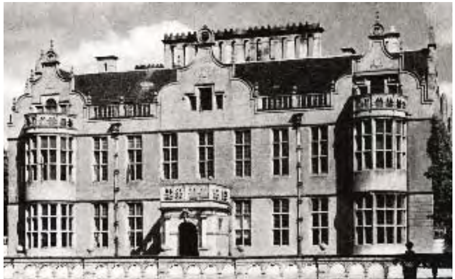
68. Lilford Hall, Northamptonshire, 1635, south front showing stepped 'Venetian' windows in the gables. (Ralph Dutton, The English Country House , 1935)
